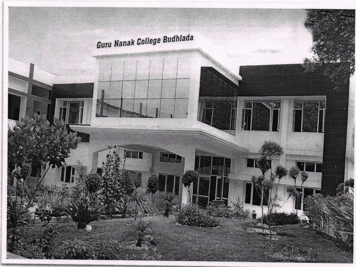
View of Administrative Block
