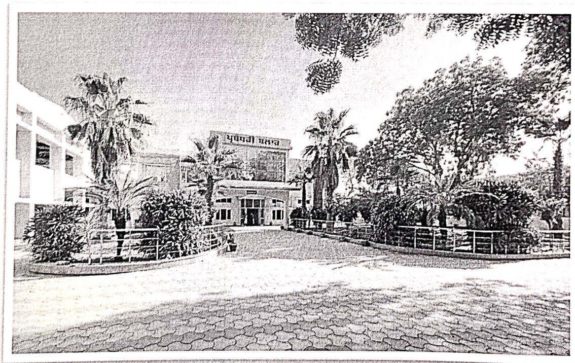
View of Administrative Block
