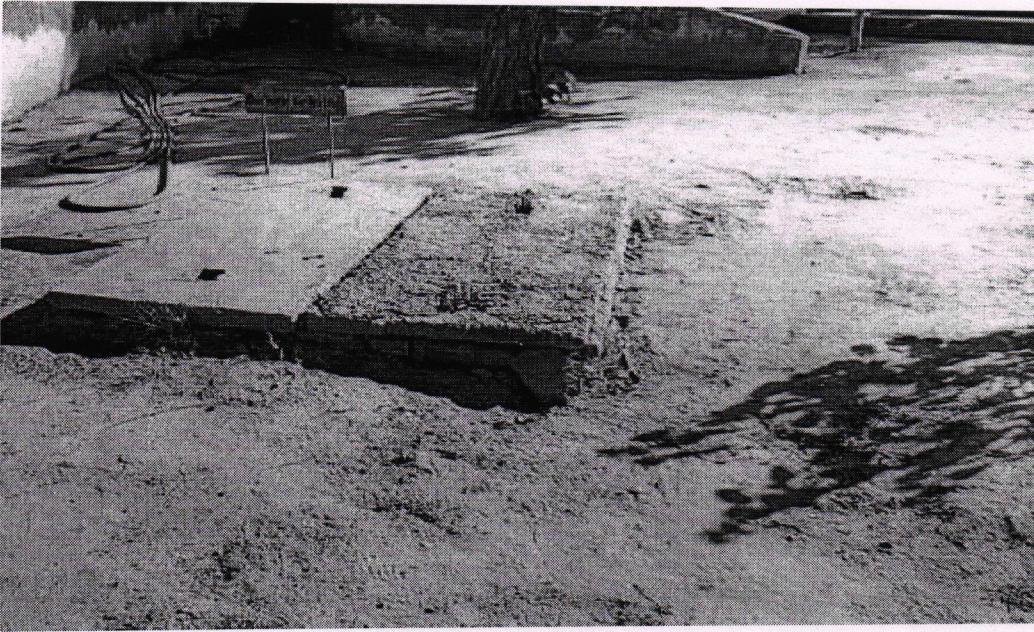
Rainwater collection tank
