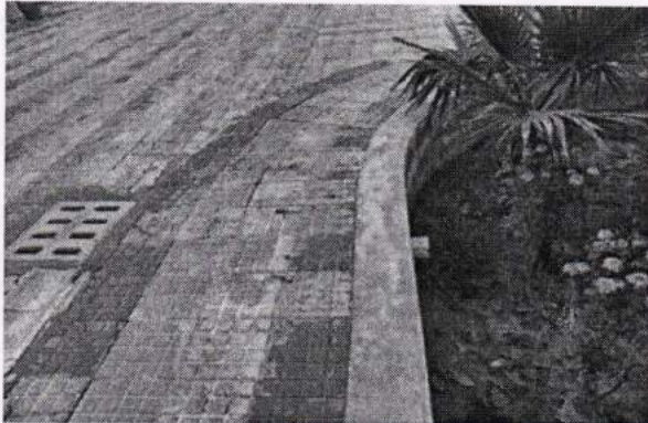
Floor Water discharge in lawn
