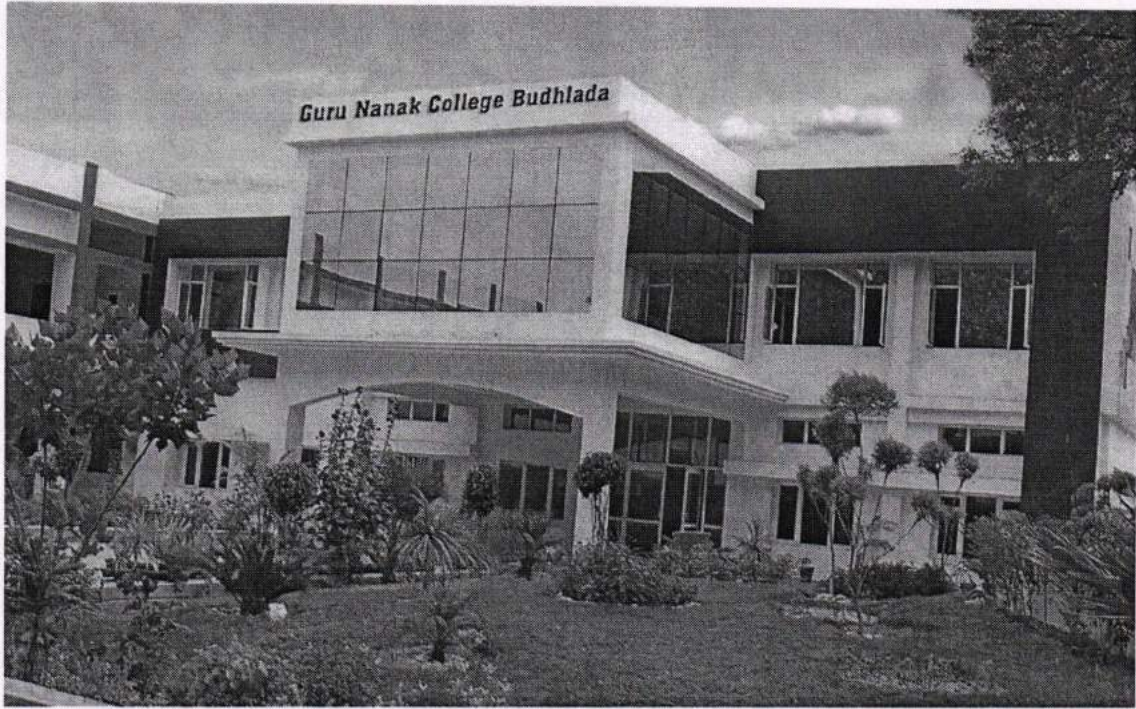
Overview of Administrative block
